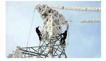
Fig. 15 Icing of transmission lines.
