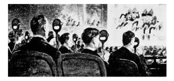
Fig. 1 Hammond's Teleview system. Only one theater in Manhattan was so equipped. Each seat in the house had attached to its back a gooseneck-mounted spinning mechanical shutter which was run in synchrony with the projector shutters. This is the precursor of all field-sequential movie and TV displays which are the great majority of products on the market.
