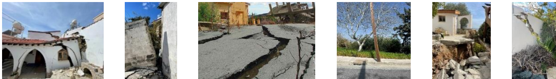
Figure 1: Photos showcasing the aftermath of the landslide
