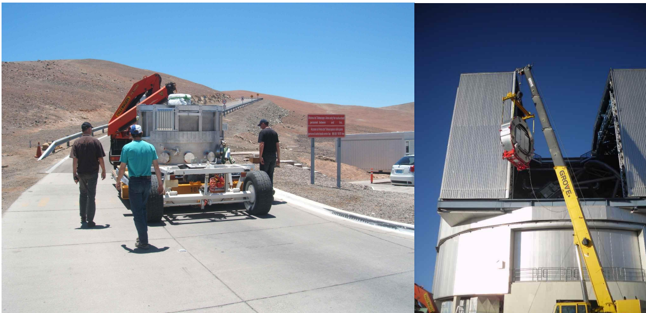
Figure 2: KMOS cryostat on the road from the integration hall to the summit (left); the CACOR being hoisted into the dome of UT1 (right).
